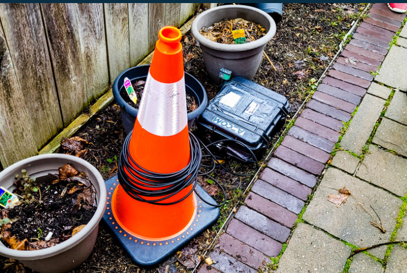
Vibration monitoring installation.
